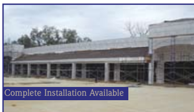
Standing Seam Metal Roofing
